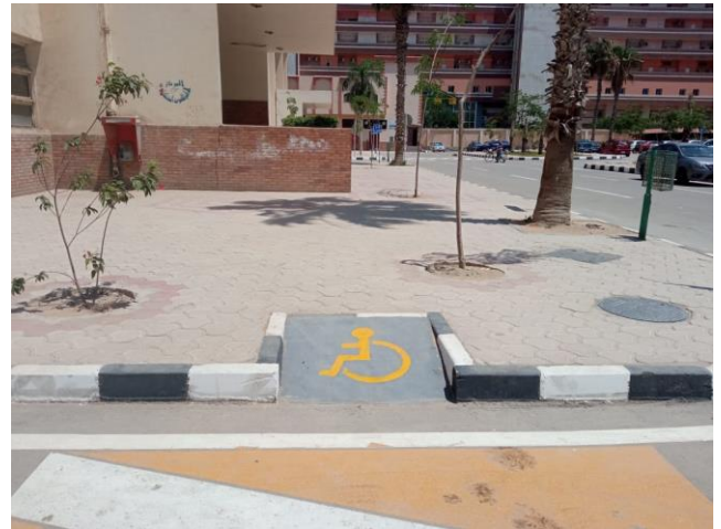
Disabled ramp (Tanta University, Egypt)
