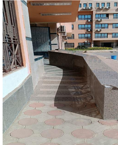
Disabled ramp (Tanta University, Egypt)
