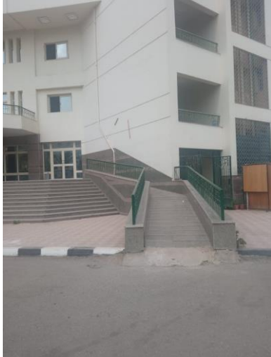
Disabled ramp (Tanta University, Egypt)
