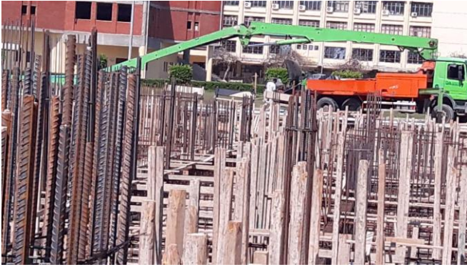
Building construction (Tanta University, Egypt)
