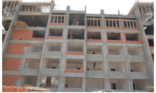
Building construction (Tanta University, Egypt)
