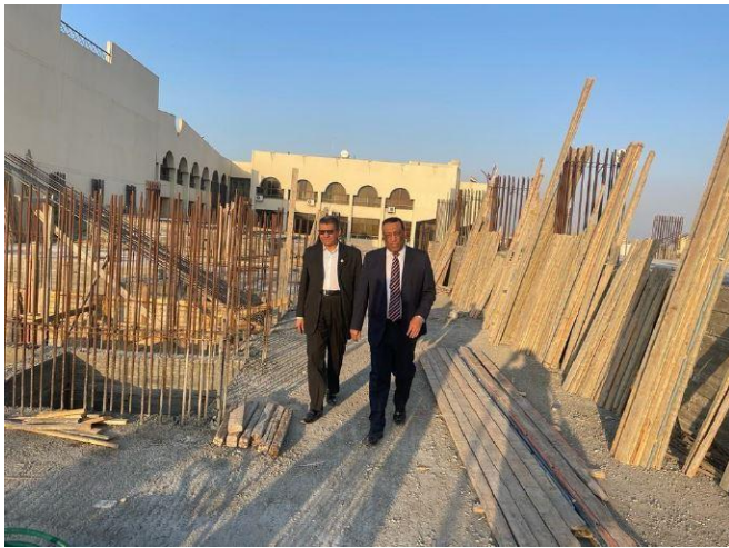
Building construction (Tanta University, Egypt)
