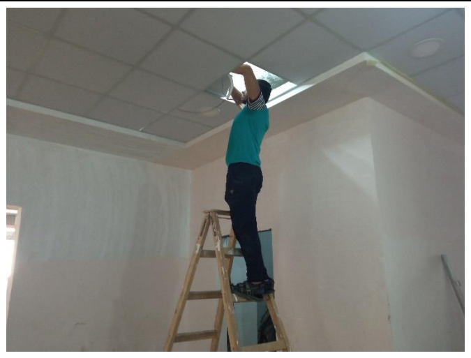
Building maintenance (Tanta University, Egypt)
