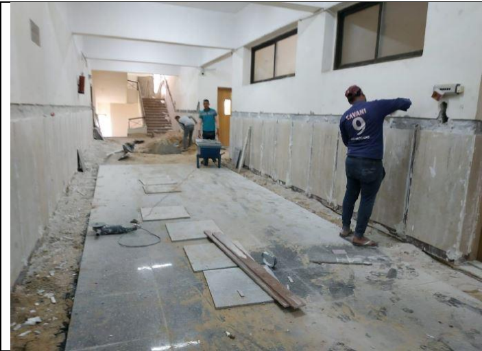
Building maintenance (Tanta University, Egypt)
