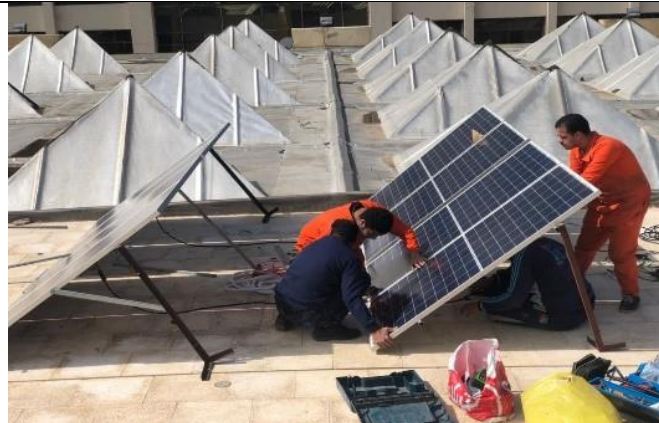
Installing Solar Panels at Sibirbay Campus (Tanta University, Egypt)
