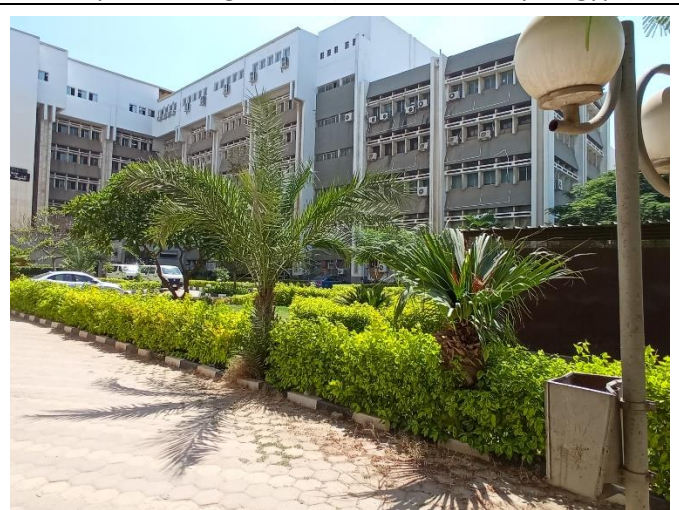
Area on campus for water absorption besides the forest and planted vegetation (Tanta University – Egypt)
